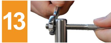
Now return to the pre-fixed cable end, using a wrench simply tighten the stainless steel nut to achieve the desired cable tension.
