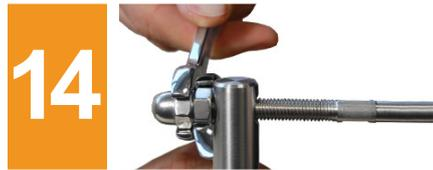
When you are happy with the cable tension, thread the dome nut on and tighten the nuts against each other.
